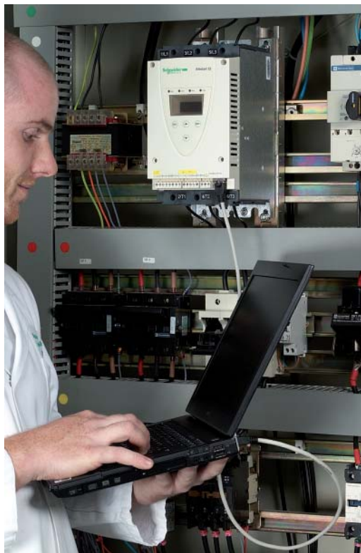
Commissioning the ATS 22 soft start - soft stop unit with SoMove lite setup software
